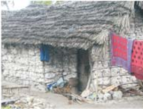
Fig. 24. Swahili house made of wood, stone, lime and coconut leaves as roofing materials Source: Field data, 2006
