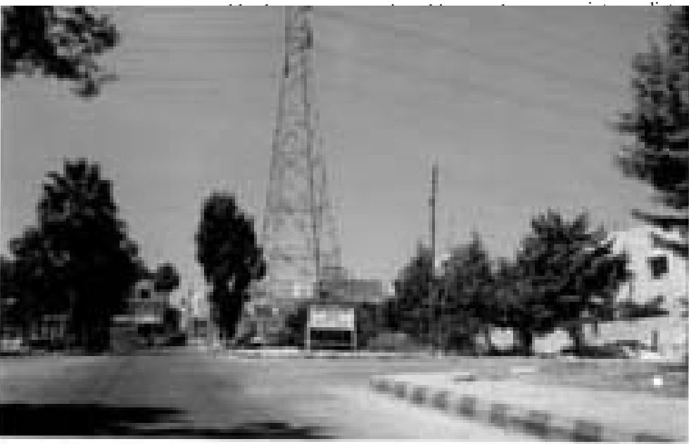
Fig. 6. The only landmark at PRH scheme, the high voltage electricity. Source: Author, 2005.
