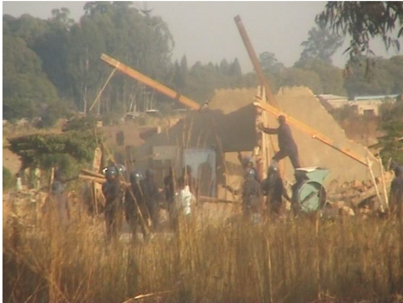
Fig. 1. Police supervised destruction of illegal structures
